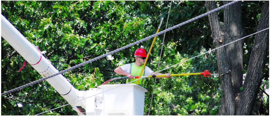
▲ An OSHA certified worker trims a tree near high-voltage lines. Special care must be taken when performing vegetation management near high-voltage power lines. Always keep at least 10 feet away from power lines. Photo courtesy of SafeElectricity.org.
