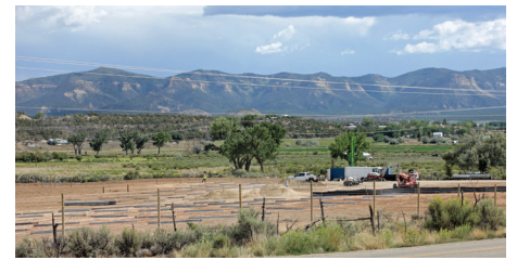
Construction on the Totten Lake solar array began in August 2020.
