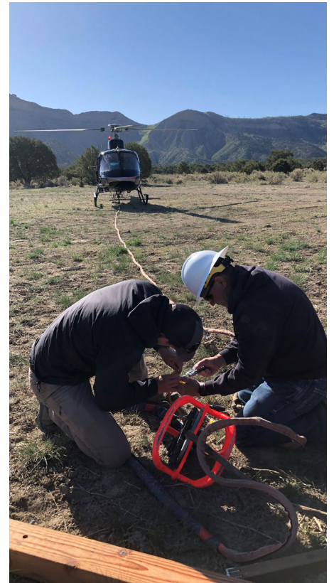
EEA's Brad Dennison (right) assists the helicopter ground crew prepare the harness used to transport poles to the job site. Photo courtesy of Orly Lucero.
