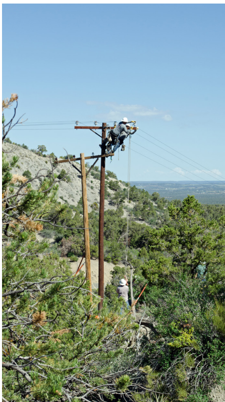
Nick Podrazik and Justin Purkat secure insulators on de-energized line with assistance from Jake Thurman and Tyler Berry. Photo courtesy of Ace Astor.
