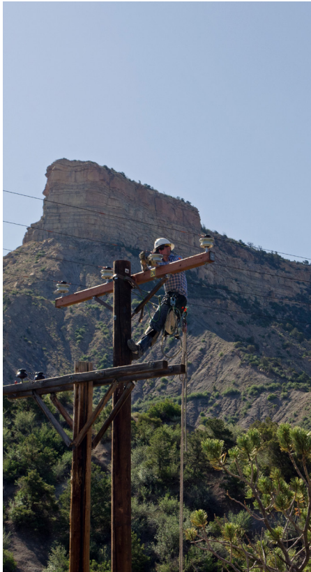
Chase Suckla attaches conductors to a new pole prior to re-energizing the line. Photo courtesy of Ace Astor.
