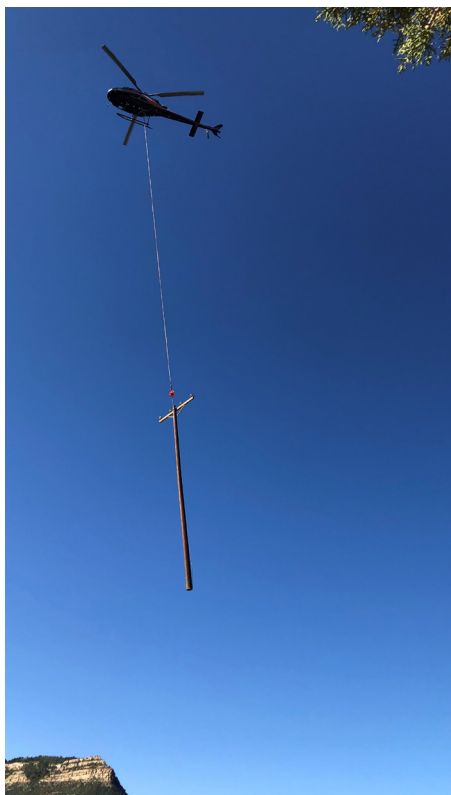
A new power pole is airlifted to the job site. Photo courtesy of Orly Lucero.
