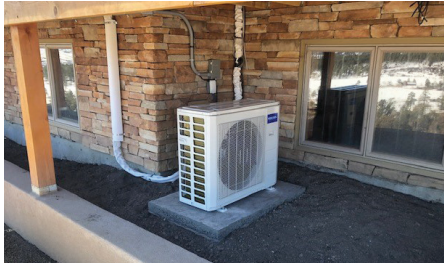
▲ Air-source heat pumps are a good option for energy-efficient summer cooling.
