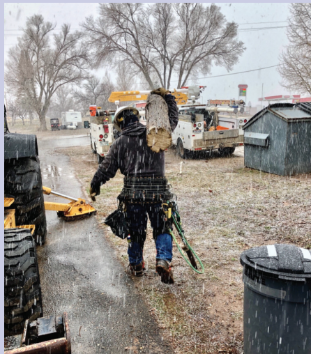
▲ EEA Lineman R.L. Wilcox removes a damaged pole section during an outage.
