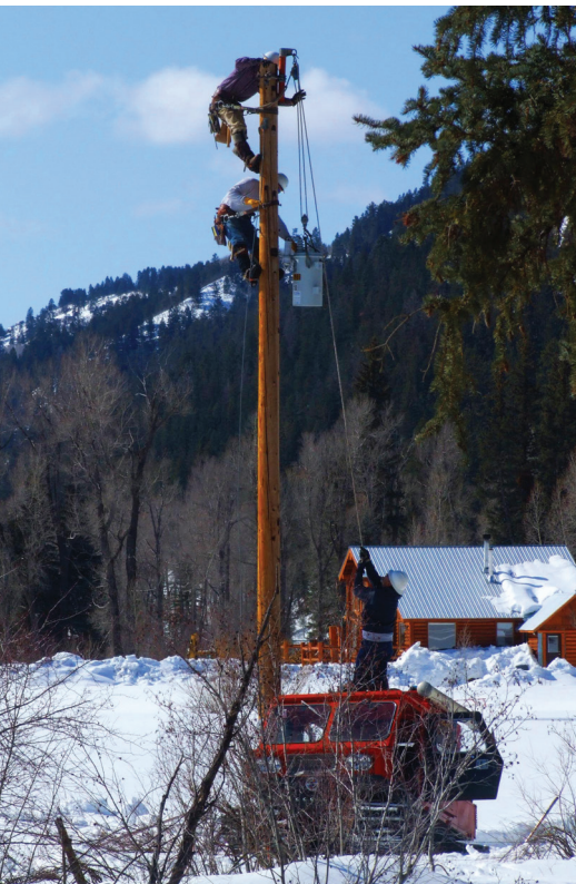
▲ EEA Lineman R.L. Wilcox removes a damaged pole section during an outage.
