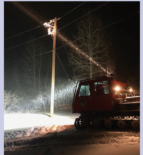
▲ An EEA line crew works an outage using a snow cat during a winter storm.
